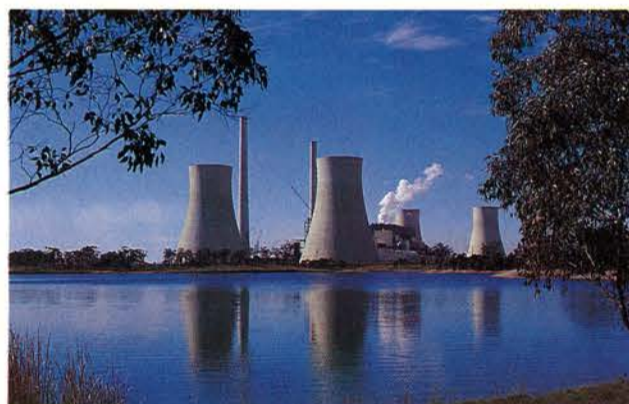
Large thermal power stations have been constructed in the upper Hunter valley in New South Wales, where there are extensive deposits of black coal. This photograph shows the 2640-megawatt Bayswater power station in its final stages of construction. The plume of steam in the background is from the 2000-megawatt Liddell power station. Water to cool the thermal generators of both Bayswater and Liddell comes from the artificial Lake Liddell, fed by the Hunter River, and by water diverted from the upper reaches of the Barnard River, a tributary of the Manning. ELECTRICITY COMMISSION OF NEW SOUTH WALES
